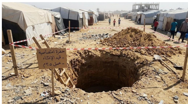
Figure 3: Unlined pits are the simplest and quickest type of cesspit constructed in the Gaza Strip, especially in temporary displacement areas
