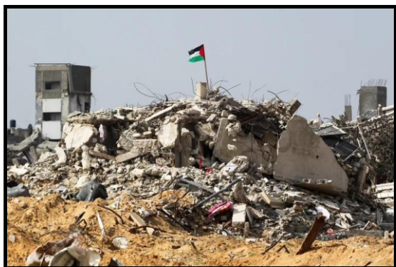
Figure 1: Rubble and collapsed buildings resulting from the ongoing Israeli War of Genocide and Ethnic Cleansing (2023–2026) in the Gaza Strip provide ideal refuges for rodents, reptiles, and other pest species.
