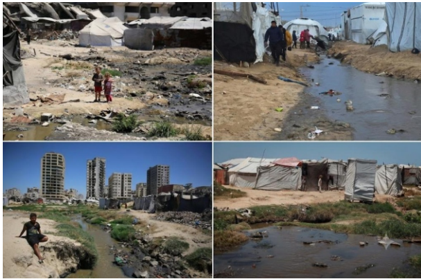
Figure 4: Untreated sewage discharge and standing water resulting from damaged sanitation and drainage infrastructure in Gaza displacement camps
